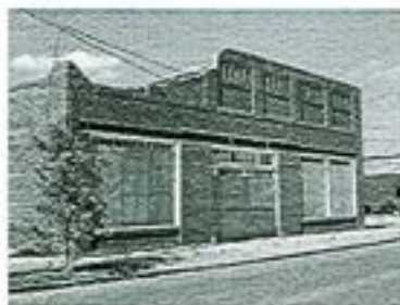
Existing Feed Store Building
